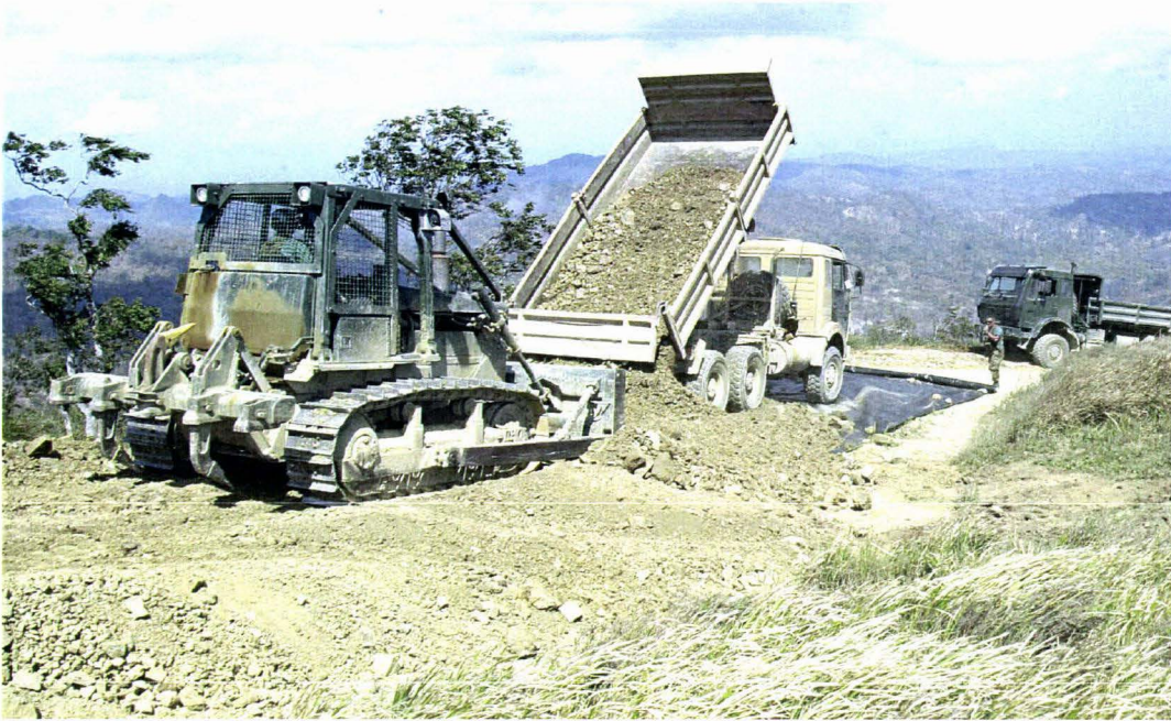
Plate 1. NZDF engineers maintaining roads in Cova Lima. (Photo NZDF)
