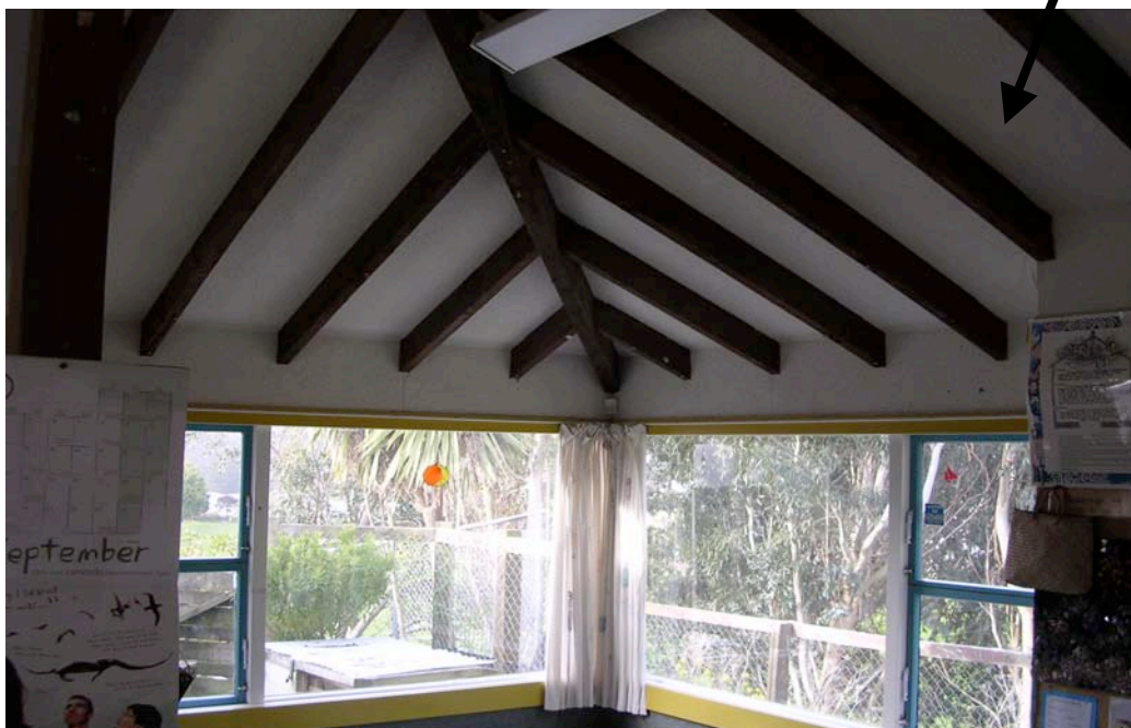
Figure 10-2 Purpose built early childhood centre. (The ceiling and upper wall to top of window sills coated with asbestos containing textured finish).
