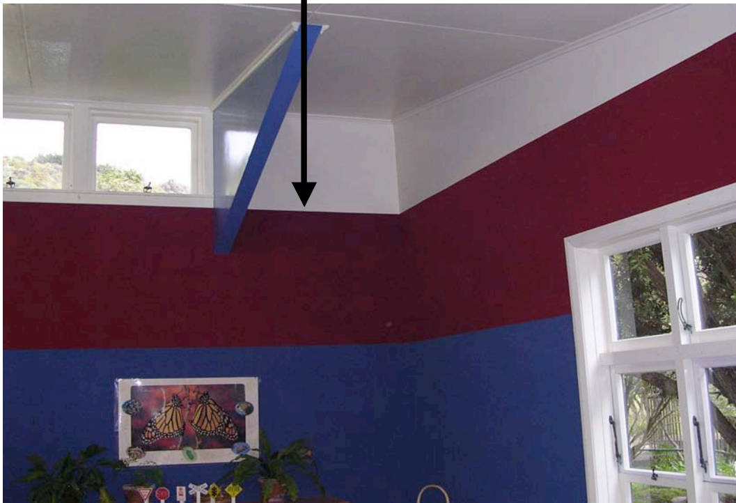
Figure 10-4 Acoustic wall treatment to the upper window sill Case 1
