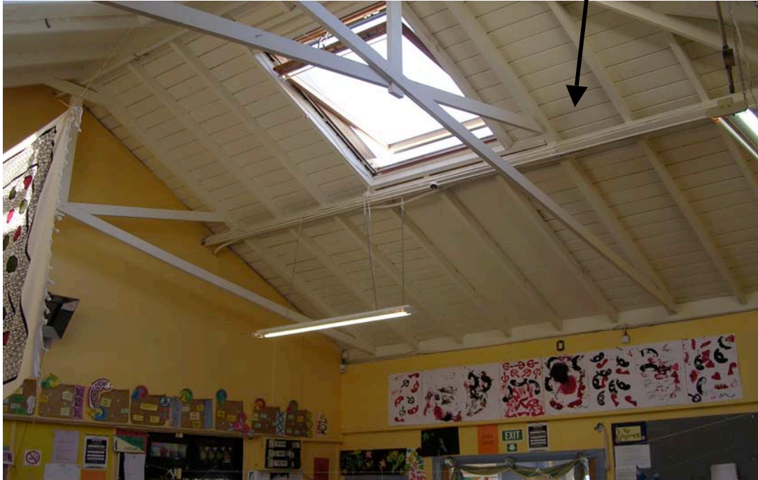
Figure 10-1 An all day centre showing a pitched ceiling (with exposed sarking over rafters) and presence of skylights.
