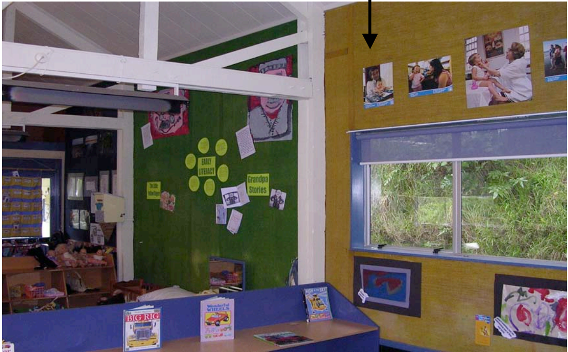
Figure 10-7 Walls lined with hessian surfaced soft board panels Case 3
