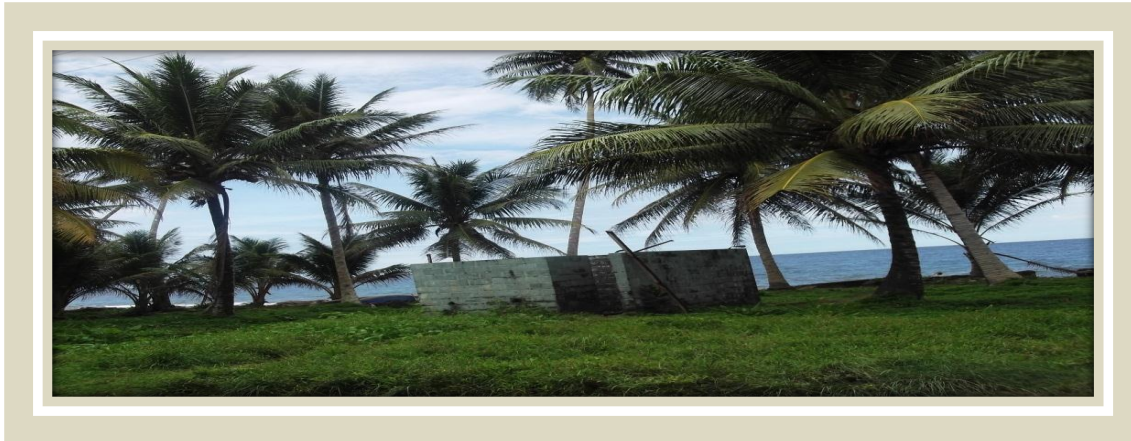
Figure 7.1: An abandoned ablution block in Narian Village, Misima.
