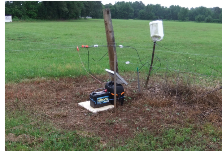
Figure 21 - B100 SP, running full power with 2.8 kV on the fence. Note no protection to stop cattle knocking over or removing the Alligator clips.
