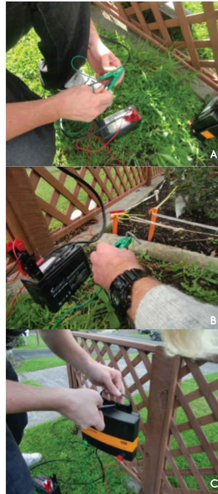
Figure 30. A) Attaching wire into crocodile clip. B) Connecting energizer grounding cable to the grounding rod. C) Participant is unsure what to do with grounding rod
