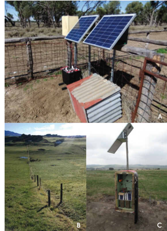
Figure 34. A) Large solar setup in Australia. B) Typical NZ farm. C) Permanent system setup in an old fridge.
