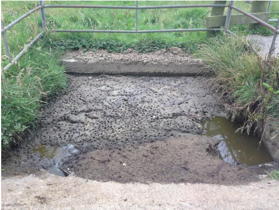
Figure 3.1. Image taken of the wedge (sand-trap) as part of the effluent system on a Waikato dairy farm. Photo provided by LIC.
