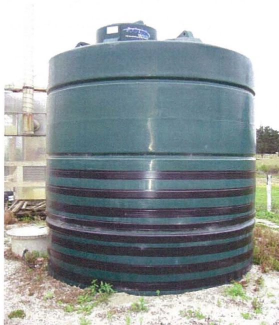
Figure 4.2.5 Slow sand filter tank
