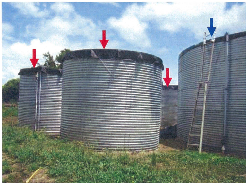
Figure 4.1.4 Reused nutrient solution storage tanks (red arrow) and raw water storage tank (blue arrow).
