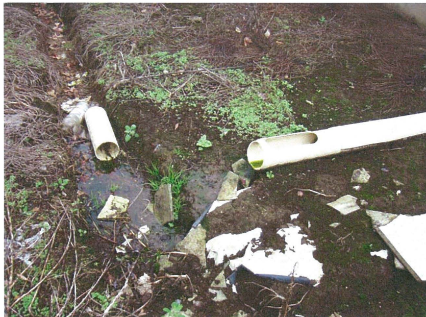
Figure 4.3.4 The nutrient solution drainage is guided to the open land out of the greenhouse through a pipe.
