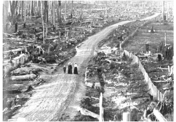
Mangahei after a fire (CS Kilford) Dannevirke Museum
