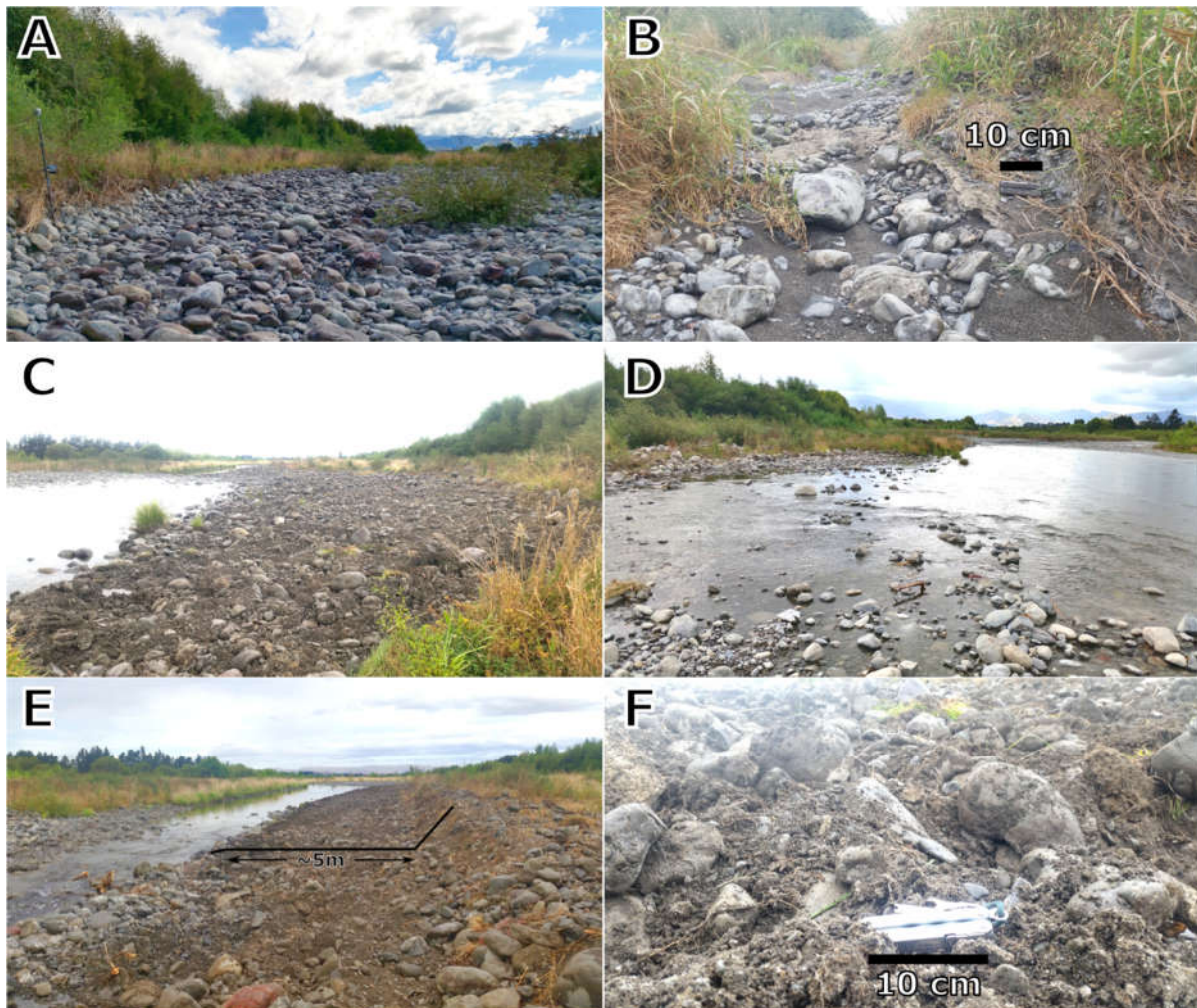
Figure 7-12. Selected examples of substrate characteristics in the segment AOI. A: A mature (though still mobile) bed armor layer. B: floodplain channel prior to flow augmentation from channel realignment C and D: Vicinity of STA 9+50 where inlet capacity of floodplain channel was increased C: as-built condition on 2019-02-21 looking downstream following armor removal and excavation (directed to B) D: same location looking upstream two days later following the first freshet (57.9 cumec peak). Total discharge (distributed across all channels) in the second photo is approximately 5 cumecs greater, but considerable reworking and winnowing has already begun. E: As-built conditions in a gravel extraction zone (material source for bank groynes) to enlarge channel capacity (E) and close-up of grain size distribution (F) from the inlet area shown in C and D.
