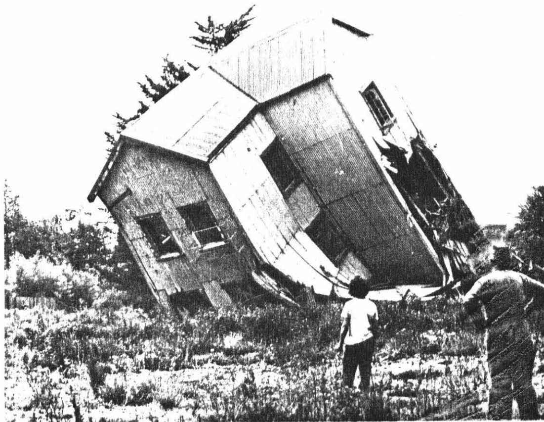
Plate 17 The demolition of Flemings Mill. (Source: Christchurch Press Co. Ltd. )
