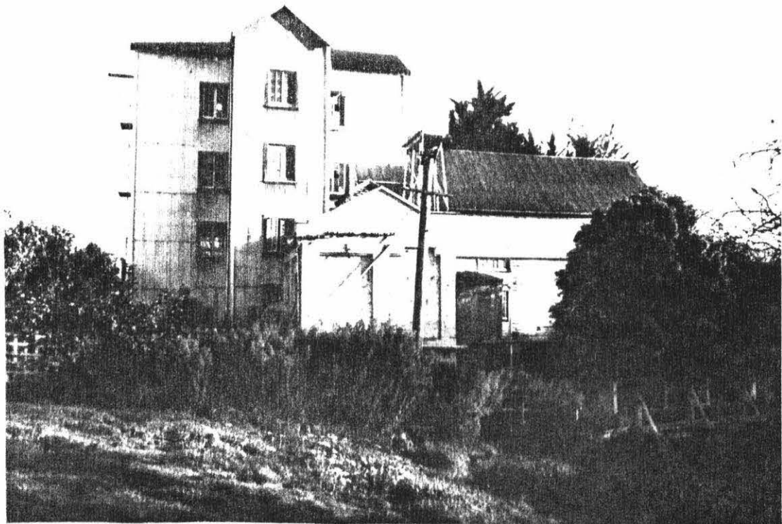
Plate 16 Flemings Mill, Christchurch. (Source: The New Zealand Newspapers Ltd., Christchurch.)
