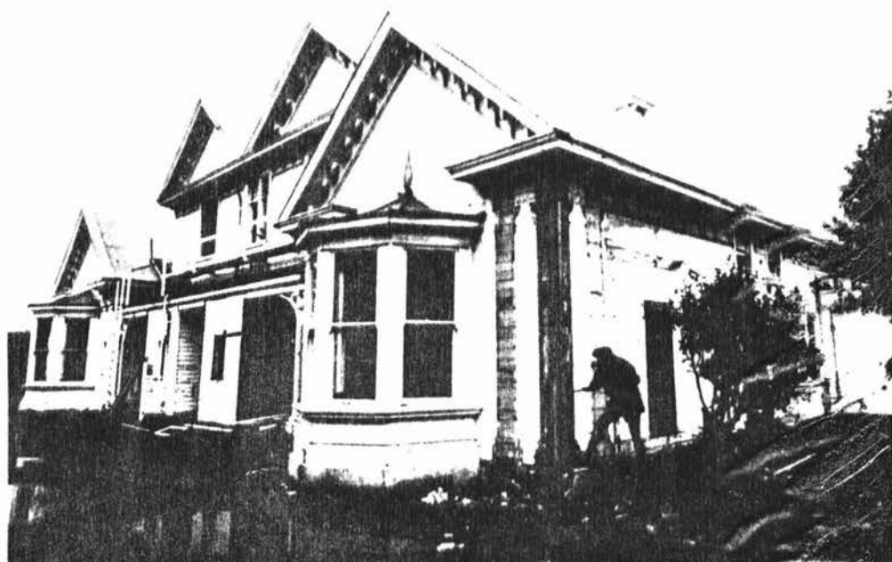
Plate 8 The Demolition of Sandridge Hall. (Source: Wanganui Newspapers Ltd.)
