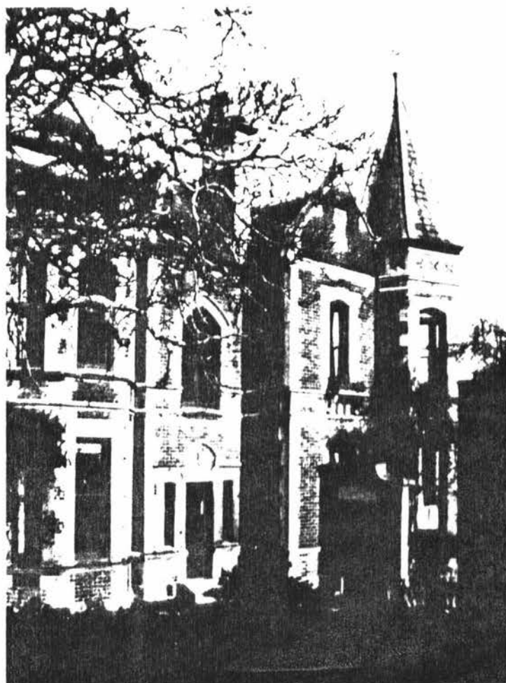
Plate 23 The somewhat eerie gothic structure of the Knox Church Manse, Dunedin. (Source: Otago Regional Committee of the Historic Places Trust.)
