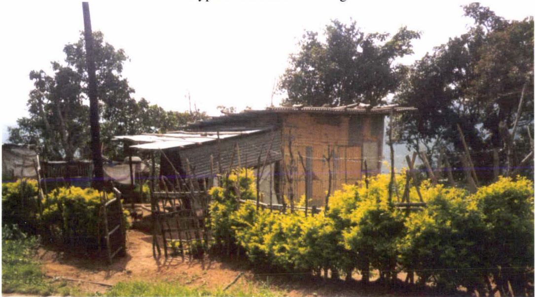
A typical house is made of galvanized iron roof and wooden planks for walls.
