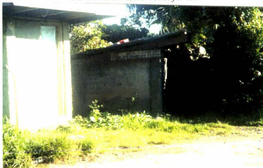
Figure 7.14 CIDSS-constructed Toilet for All
