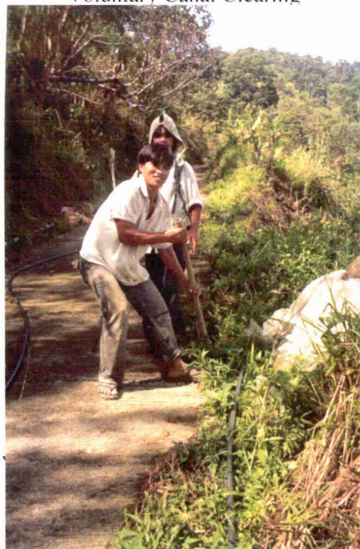
Figure 8.28 Voluntary Canal Clearing
