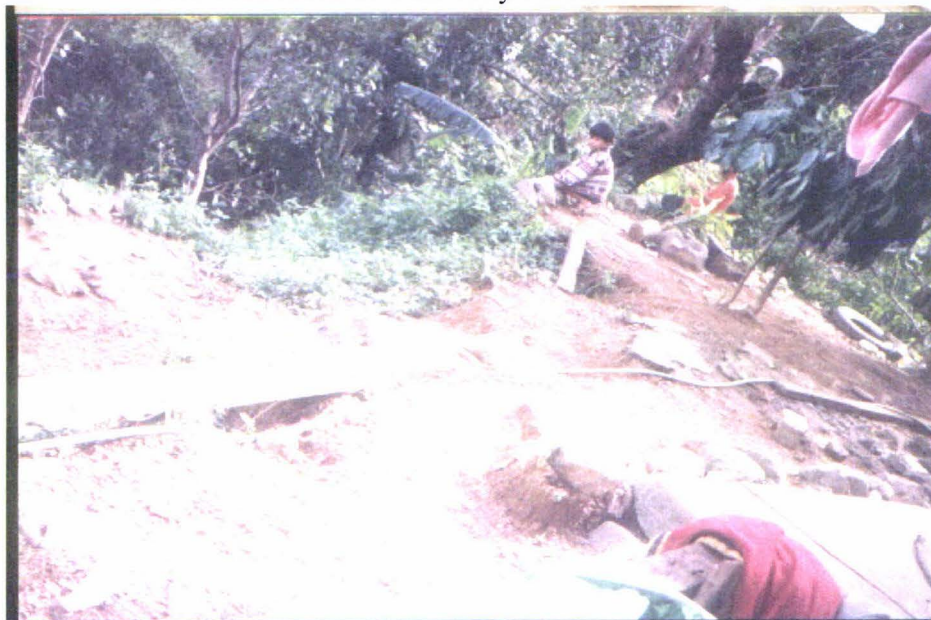
Figure 8.3 63 Transformation of the Peday Farm to Market Road
