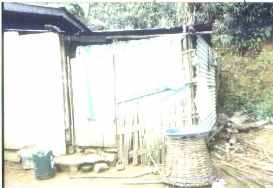
Figure 8.6 Galvanised Iron Sheets Provided by CIDSS for House Repair
