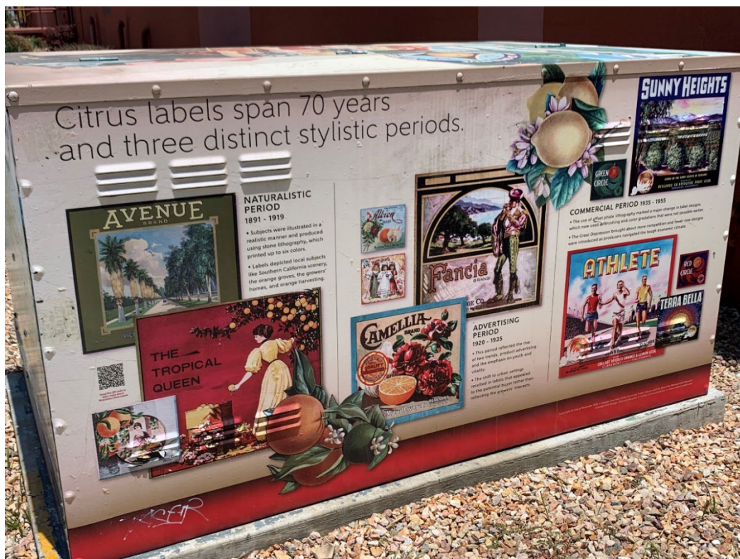
Figure 6.8: A history of citrus labels displayed on an electrical service box. Photo taken by author in 2023.
