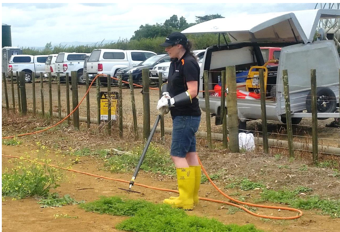
Figure 1-4 Photograph of the Rootwave Pro™ system by HotGrass Ltd. At a Pukekohe, NZ demonstration of showing the treatment electrode, heavy duty electric cable, trailer with generator, and operator wearing electrically tested insulating gloves and footwear.
