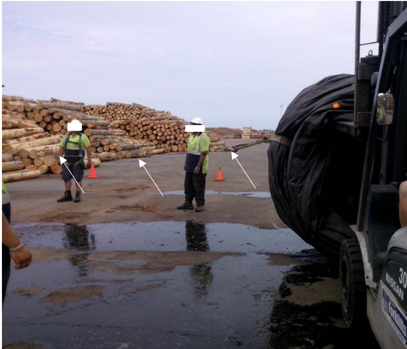
Figure 2.11 Tarpaulin getting rolled off with a metal rope (R. Hinz) – arrows at rope
