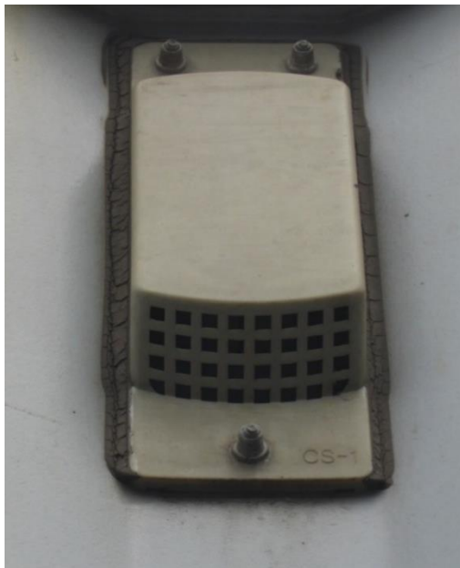
Figure 2.3 Ventilation slot (vent) outside a container (R. Hinz)
