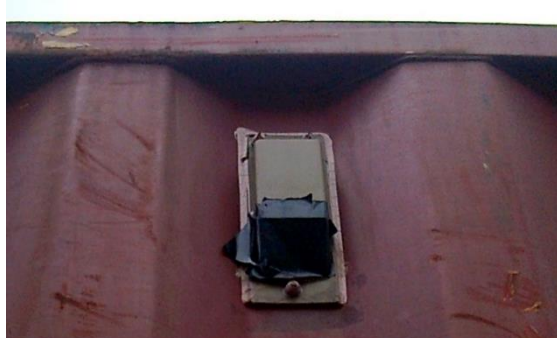
Figure 2.9 Taped vent (R. Hinz)
