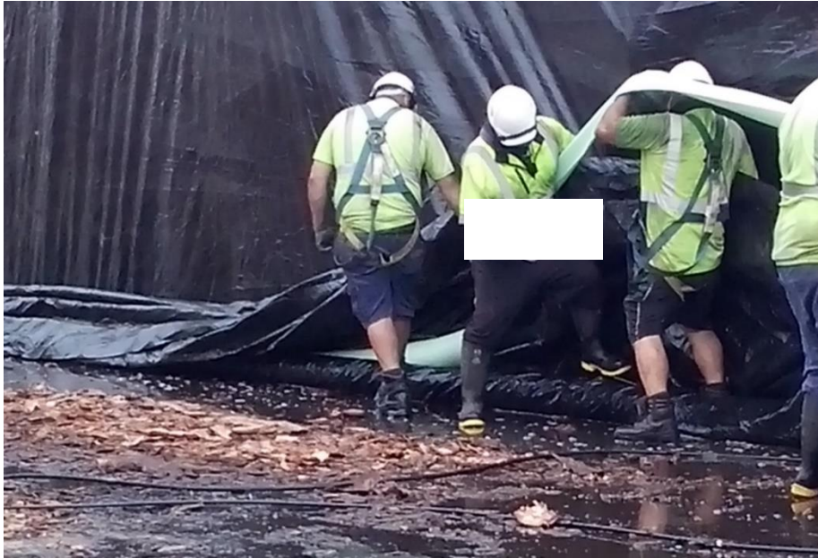
Figure 2.15 Filling and placing water snake to seal enclosure (R. Hinz)
