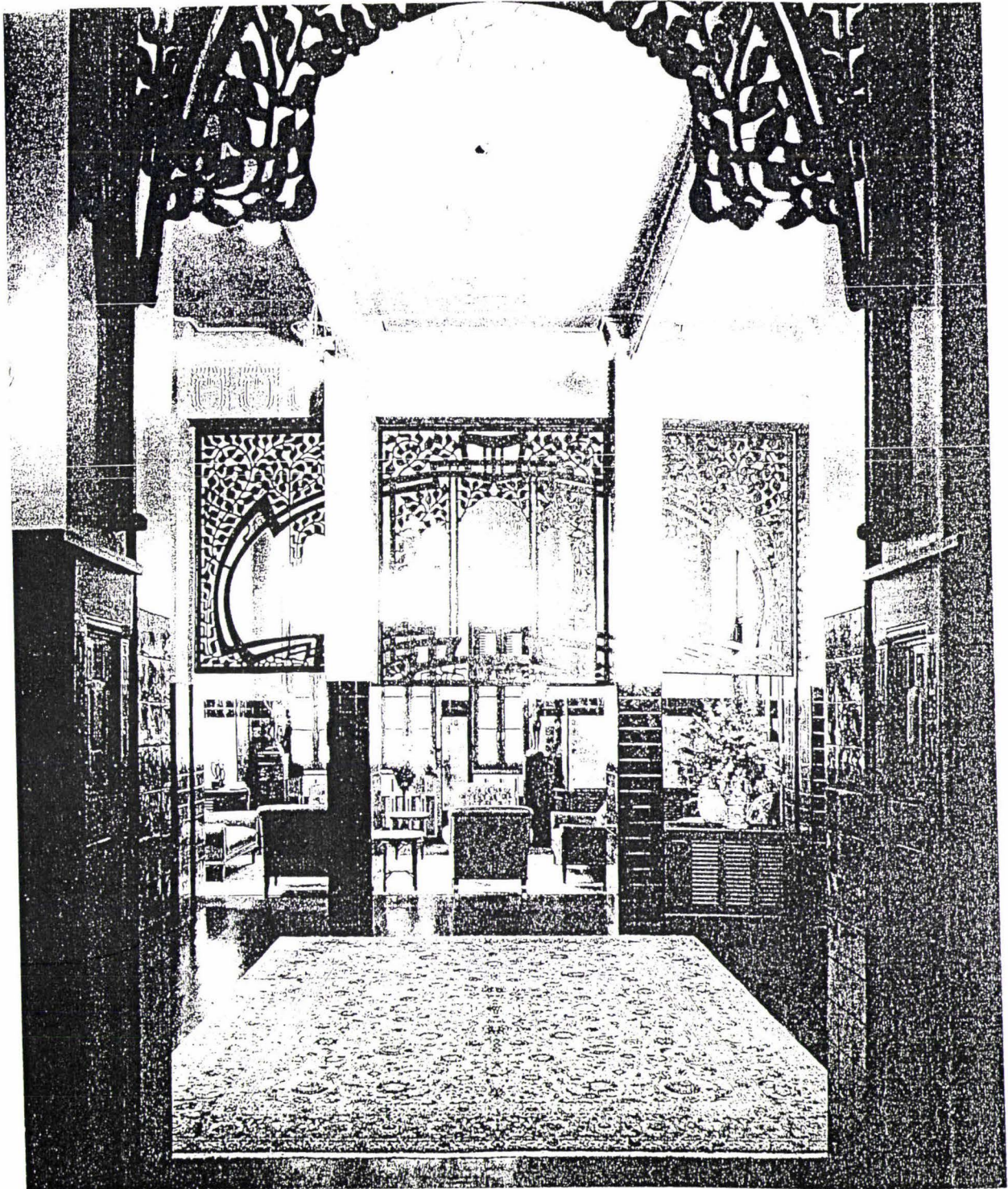
Illustration No. 4 : Another view of one of the reception rooms in the female section – Tamnak Somdaj, of Bangkhunprom Palace. Note that Art Nouveau woodcarvings above the doorways were used mainly for decorative and aesthetic purposes. These objects do not help in providing the interior spaces with good ventilation. However, they allowed the air to flow from one space to another, this also helped in balancing the overall temperature within the mansion. Even though these sitting rooms were designed without doors, in terms of spatial designs, these panels give each communal area a tangible boundary.
