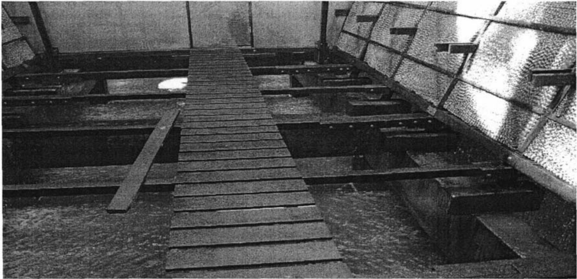
Picture 6.11: Waste Water Treatment Plant, UMC Metal Co., LTD.
