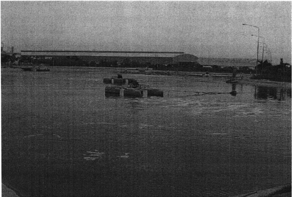
Picture 6.6: Amata Nakorn Industrial Town's Waste Water Treatment System
