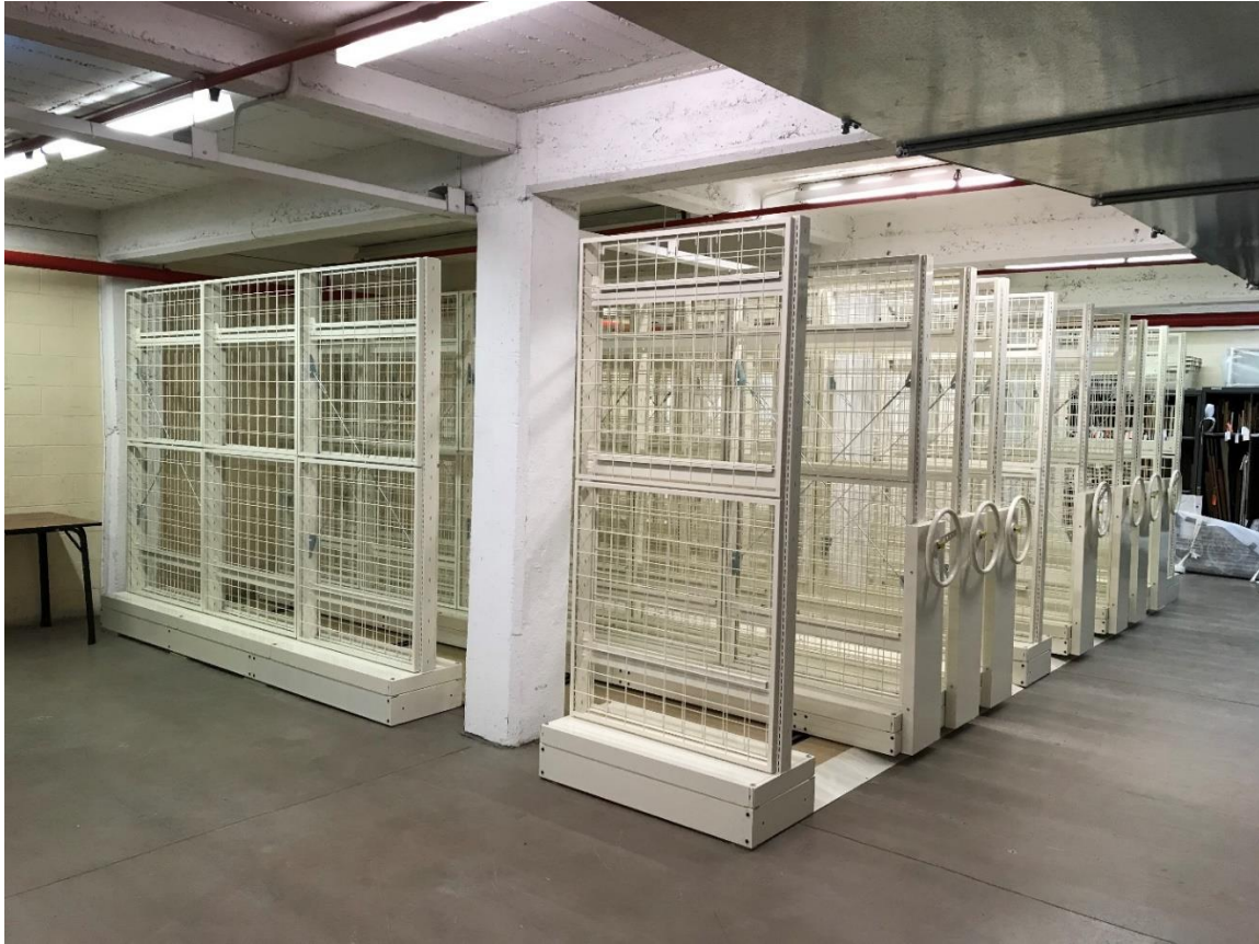
Figure 17: New rolling compactor shelving with space at either end of the room to add further rows in the future. Photograph: Author.
