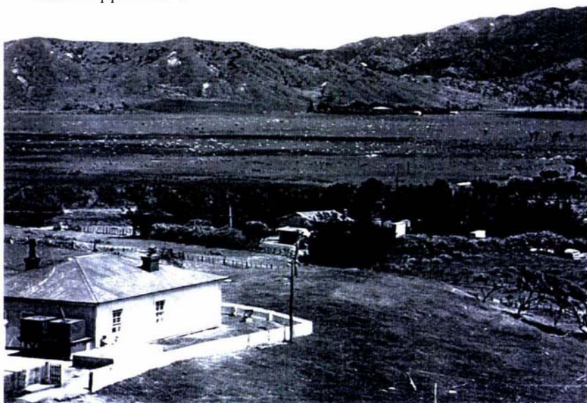
Photograph 21. East Cape 1951. The lighthouse keepers residence and East Cape School are in the foreground ( Alexander Turnbull Library: East Coast collection ).
