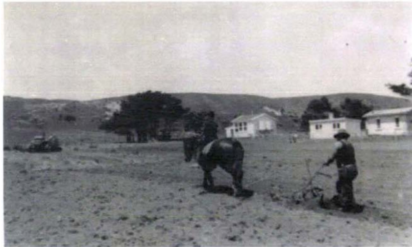
Photograph 20. Ngāti Ruawaipu have always realised that their economic future cannot be divorced from the way their people are managed. Here some of the old ways of doing things, such as scarifying, can be complementary to the use of modern machinery (such as the tractor in the background near the fence) ( Kohere collection ).
