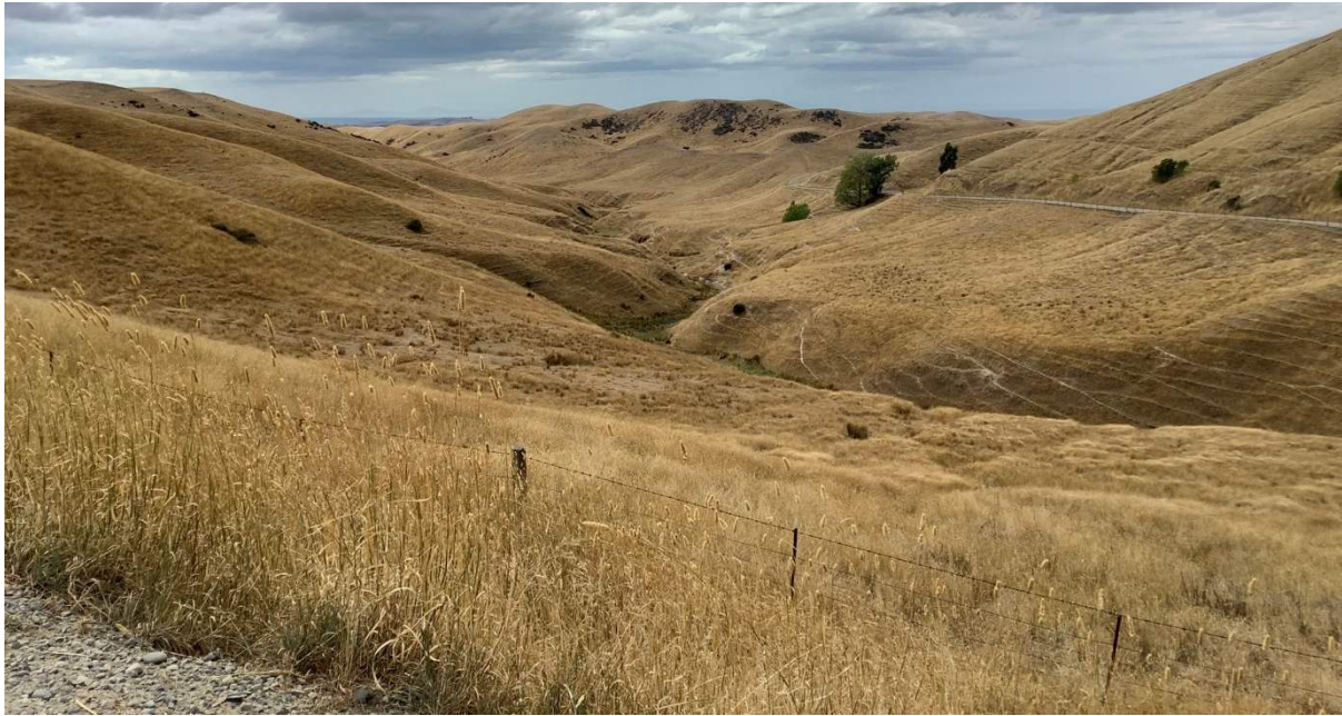
Figure 13: View from Waterfalls road looking northeast (downstream) along Nicholls Creek. Note the steep banks caused by extensive downcutting into valley fill material. Valley fill material derived from small valley side fans and slope debris.
