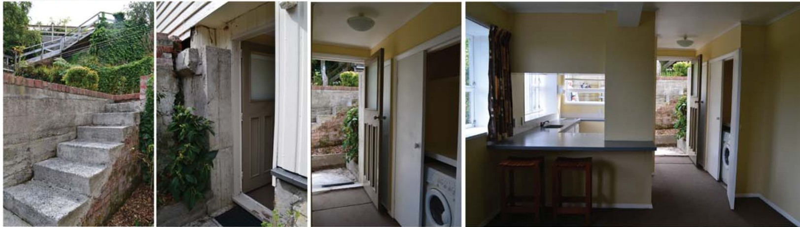
There is no internal access between the basement and ground floor.
