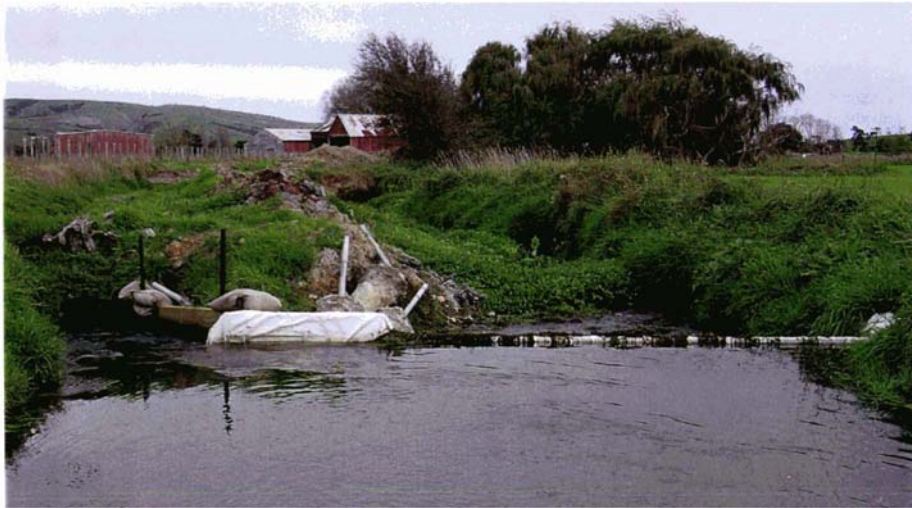
Plate 1. Weir and culvert leading to diversion channel, Booths Creek, Wairarapa.
