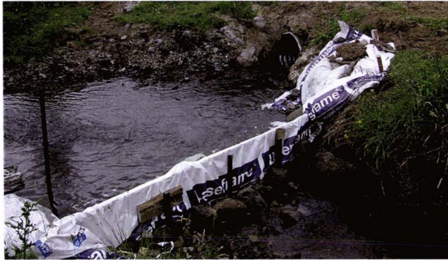
Plate 4. Weir and culvert leading to diversion channel, Kiriwhakapapa Stream, Wairarapa.
