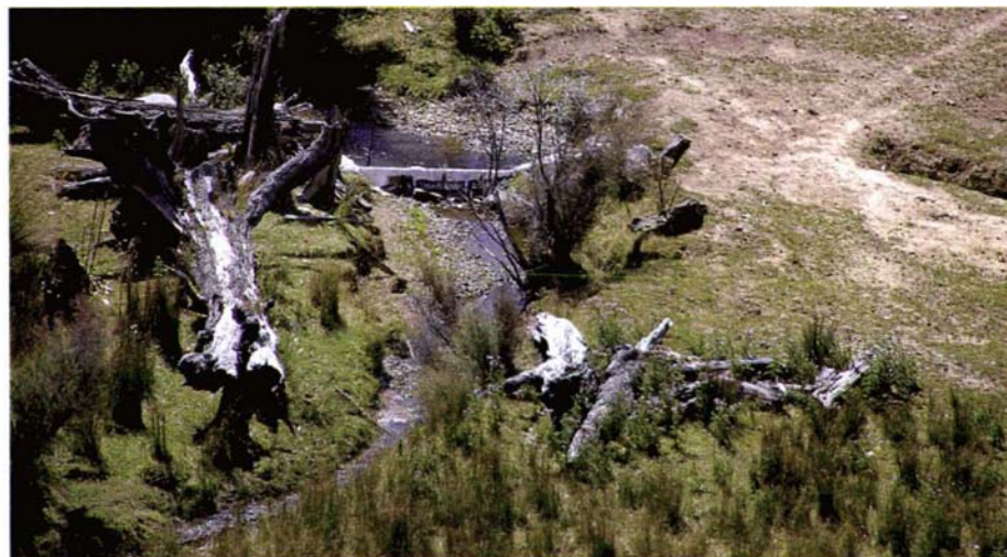
Plate 6. Weir and diversion channel (right of picture) at Kiriwhakapapa Stream.
