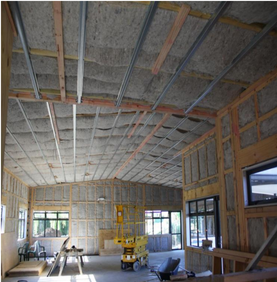
Figure 2-4 Installation of thermal insulation into a learning space
