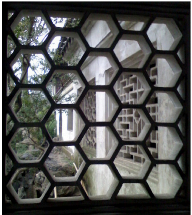
FIGURE 13 NO 2: GRID LAYOUT LEAK WINDOW DESIGN (FROM THE LINGERING GARDEN), YUCHEN XIE, 2018.
