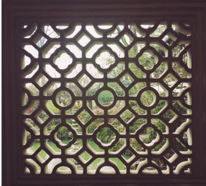
FIGURE 31: THE LINGERING GARDEN GEOMETRIC PATTERN LEAK WINDOW. PHOTOGRAPH YUCHEN XIE, 2018.
