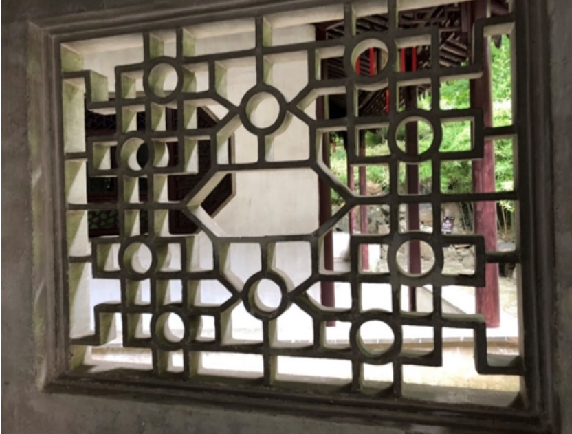
FIGURE 26: THE HUMBLE ADMINISTRATOR'S GARDEN THREE-COLUMN LEAK WINDOW. PHOTOGRAPH YUCHEN XIE, 2018.
