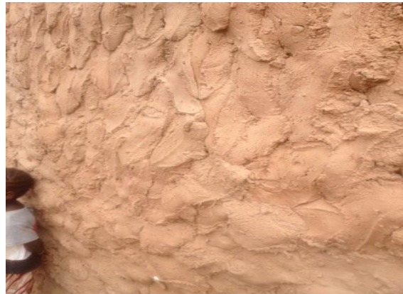
fig.4 homemade mud plaster
