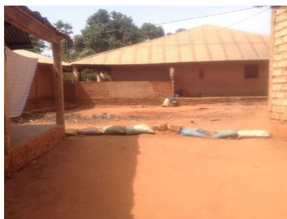
fig.2 roof: corrugated zinc sheets
