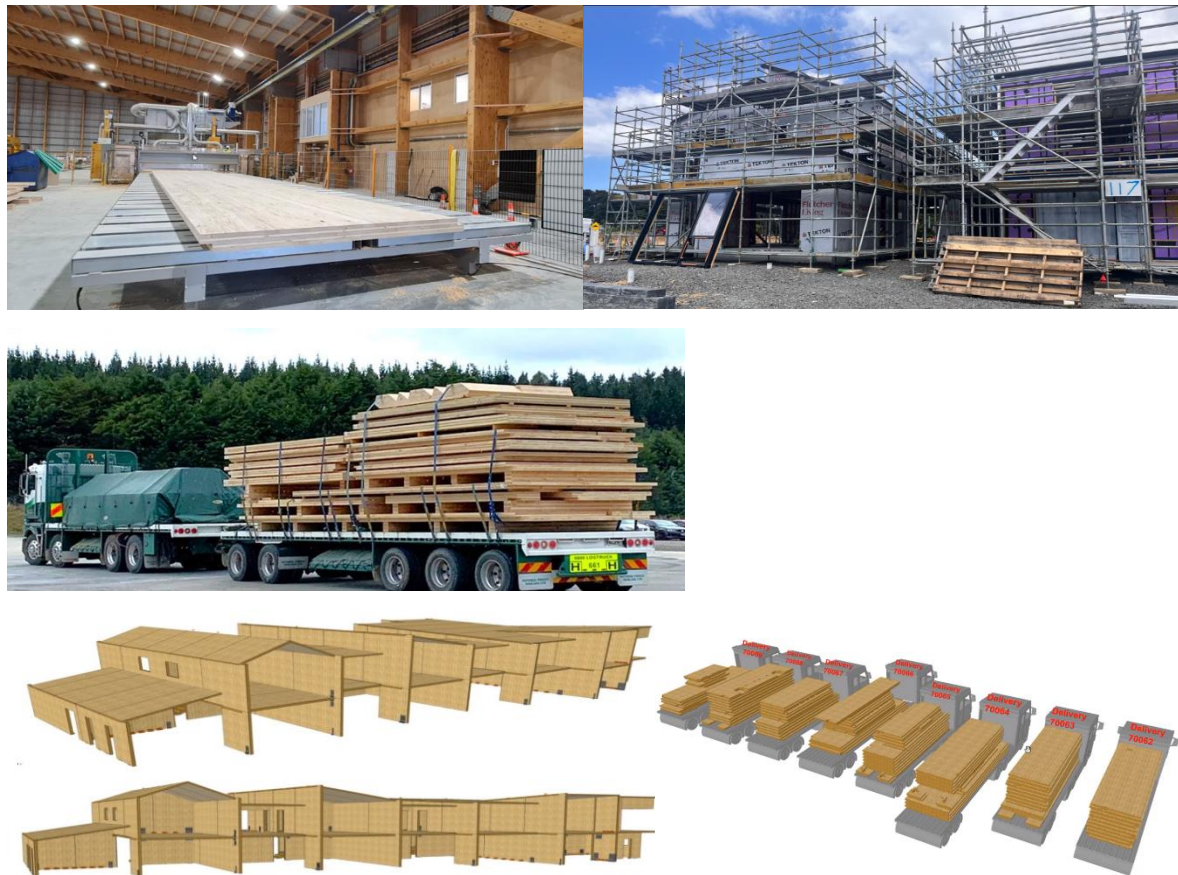
Figure 7-6: Production, Transportation and Assembly Schematics of the Panelised System.
