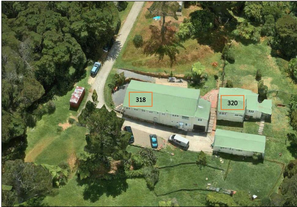
Satellite aerial view - Buildings 318, and 320.
