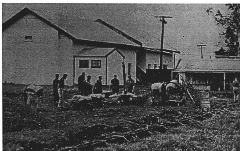
Figure 31: Foundation work for Assembly Hall, 1964.
