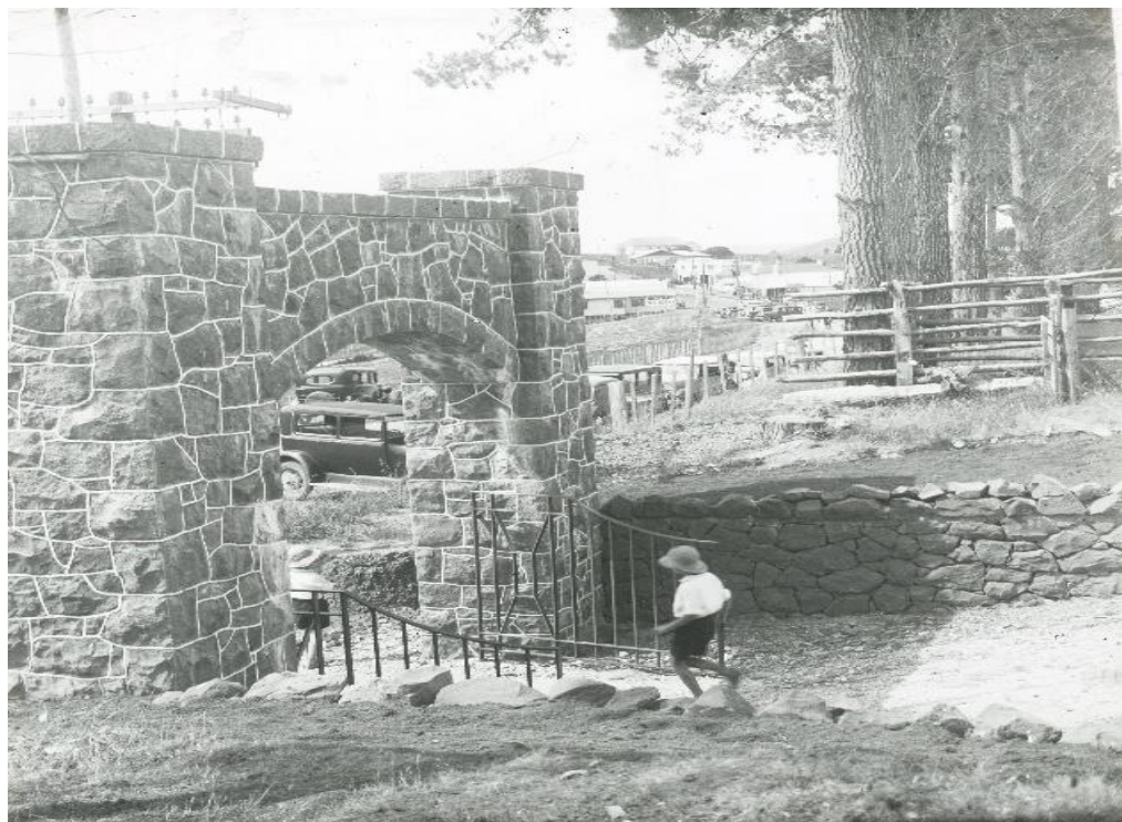
Figure 79: The Wellsford Memorial Archway shortly after its completion. Memorial Park Wellsford. Photograph, The Memorial gates , 2004.2.2007.681, Photographic Collection, Albertland & Districts Museum, Wellsford.
