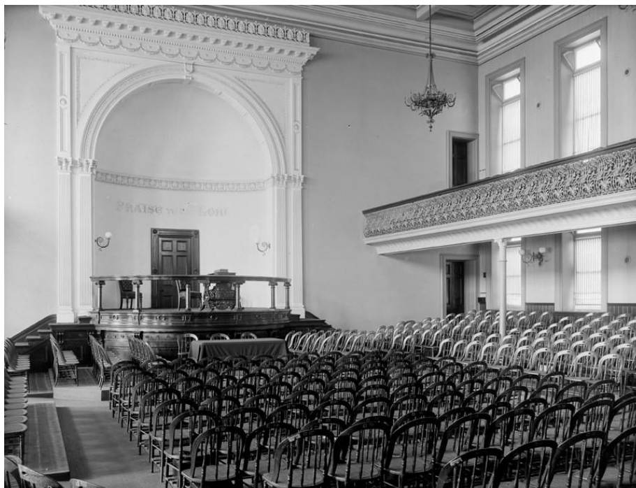
Figure 60: The Pulpit of the Auckland Baptist Tabernacle. Visible above the door are the words ‘Praise Ye Oh Lord,’ painted by Charles Blomfield with the aid of his brother Samuel. The work is now lost behind the pipe organ installed in 1913. Photograph, The Baptist Tabernacle Pulpit , “Baptist Tabernacle,” Karangahape Road, accessed 21.07.2024 https://www.karangahaperoad.com/baptist-tabernacle
