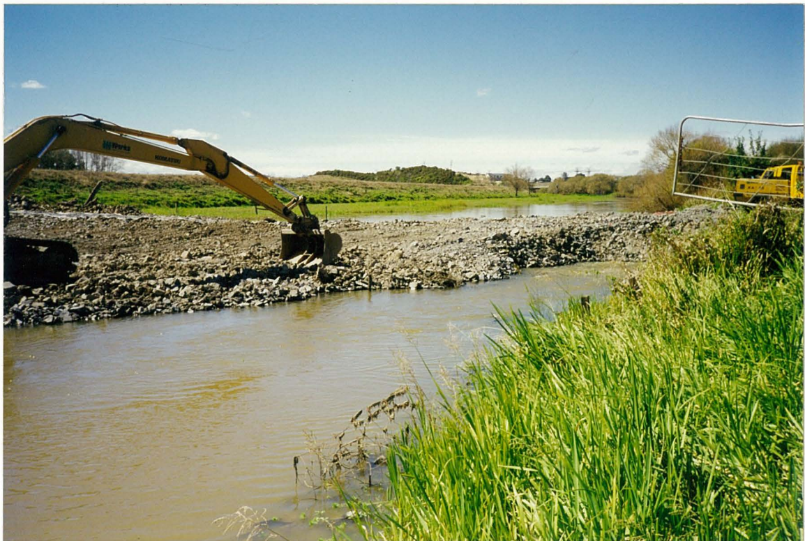
Figure 4.2 Reconstruction of the Weir - February 2000.
