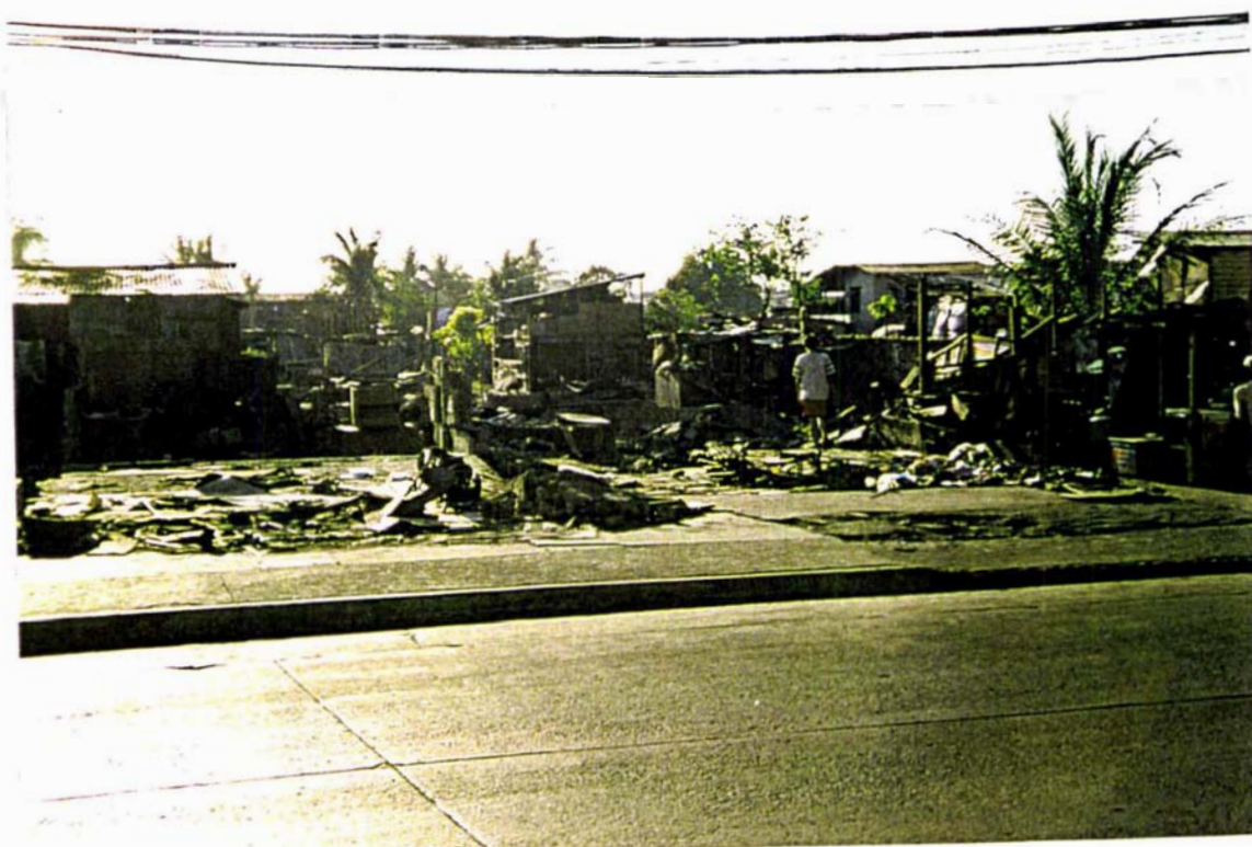
Plate 6. Demolition at dawn to make way for a shopping mall.
