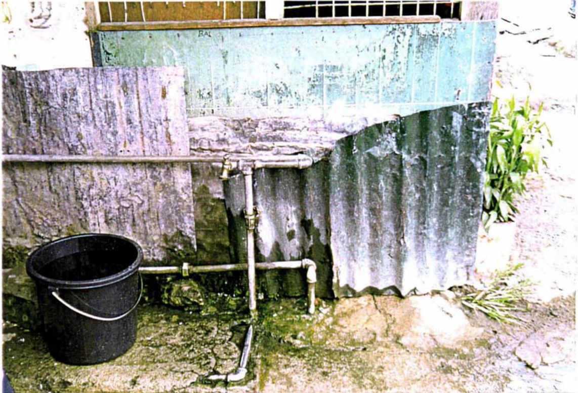
Plate 29. One of the water outlets accrued through SBT. The Chairman's house is to the left - note the personal supply line.
