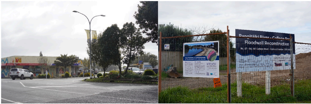
Fig. 2. Snapshots from Edgecumbe. College road (left), floodwall reconstruction site (right).
