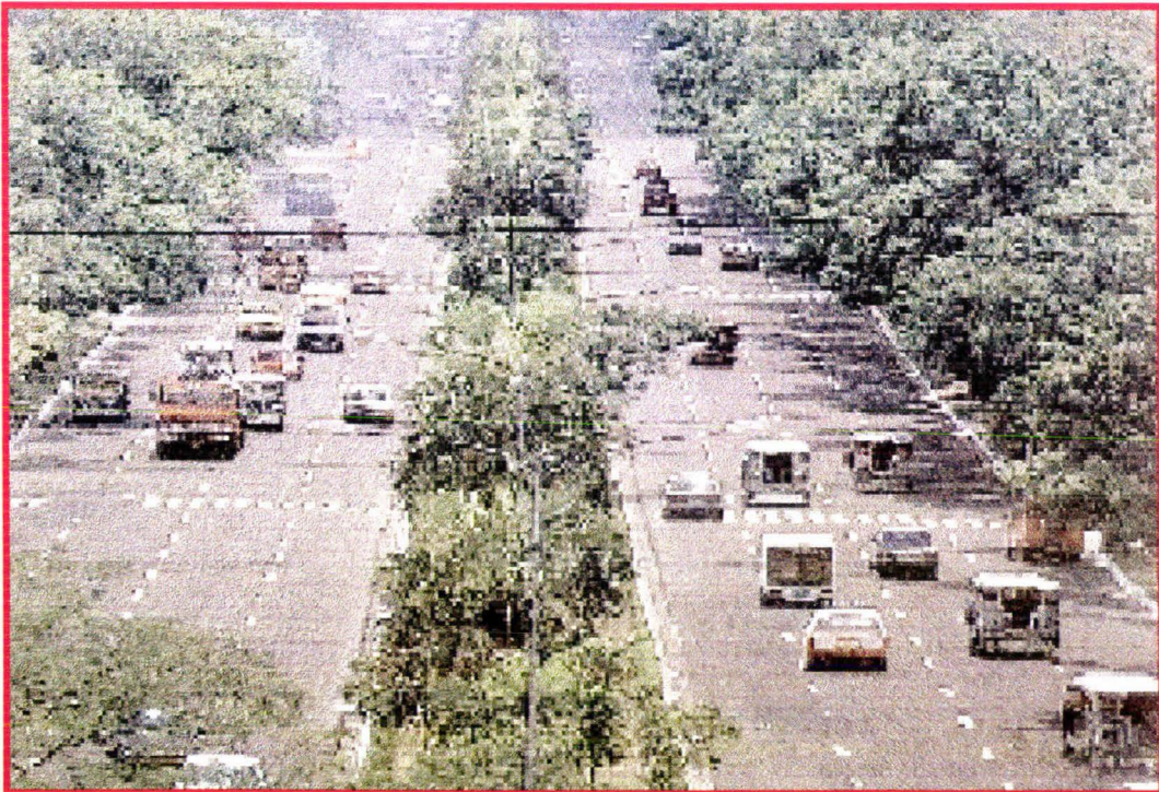
Figure 3.11. The approach to QMC and WRRC from Quezon Avenue
