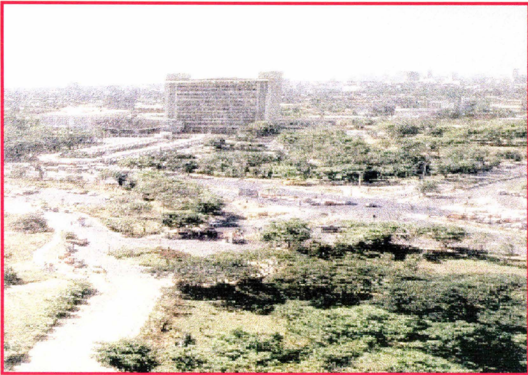
Figure 3.10. The junction between Quezon Avenue and Elliptical Road
