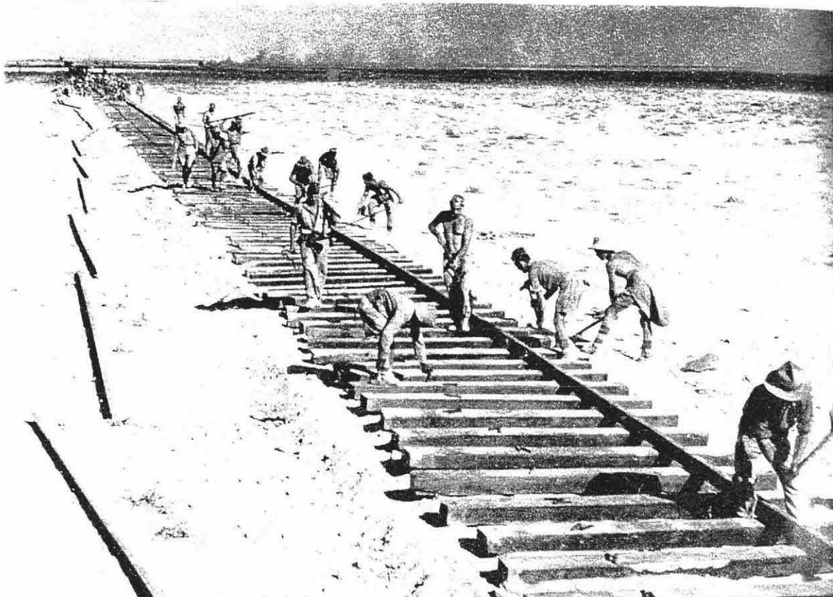
New Zealand railway construction gangs, assisted by Indian pioneer troops extending the railway in the Western Desert. New Zealand Army (M.D. Elias).
