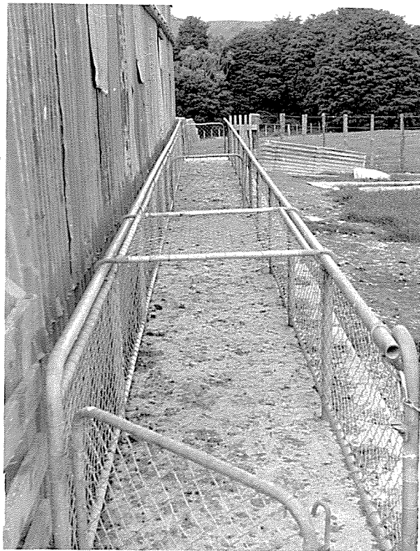
Fig. 5.2. End View of Dagging Race on Farm 49.
