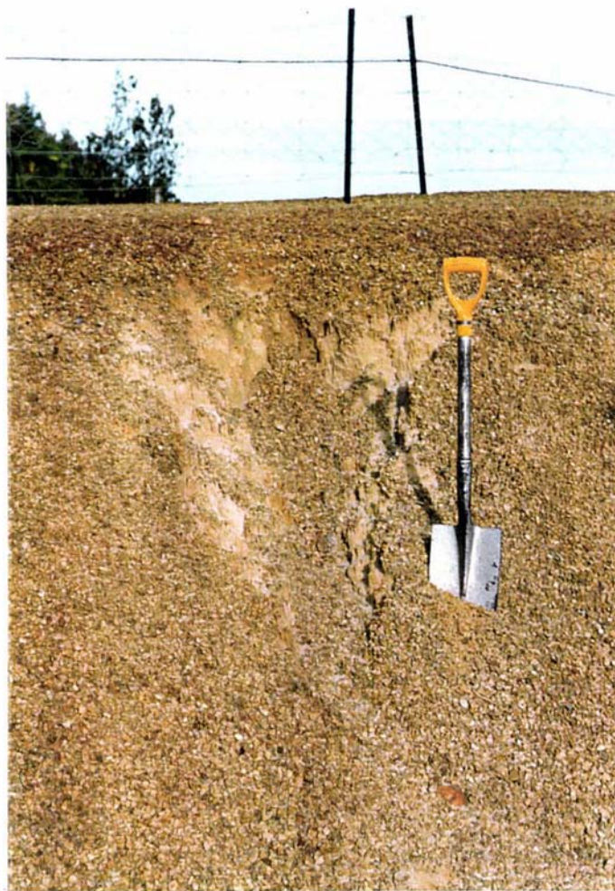
Plate 3.3 Surface erosion of Tui tailings embankment following intense rainfall (August 1993).
