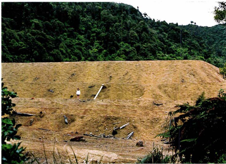
Plate 3.4 View of the front (western) face of the Tui tailings dam which is covered with a 15-20 cm layer of crushed sulphide-bearing quartz (August 1993).
