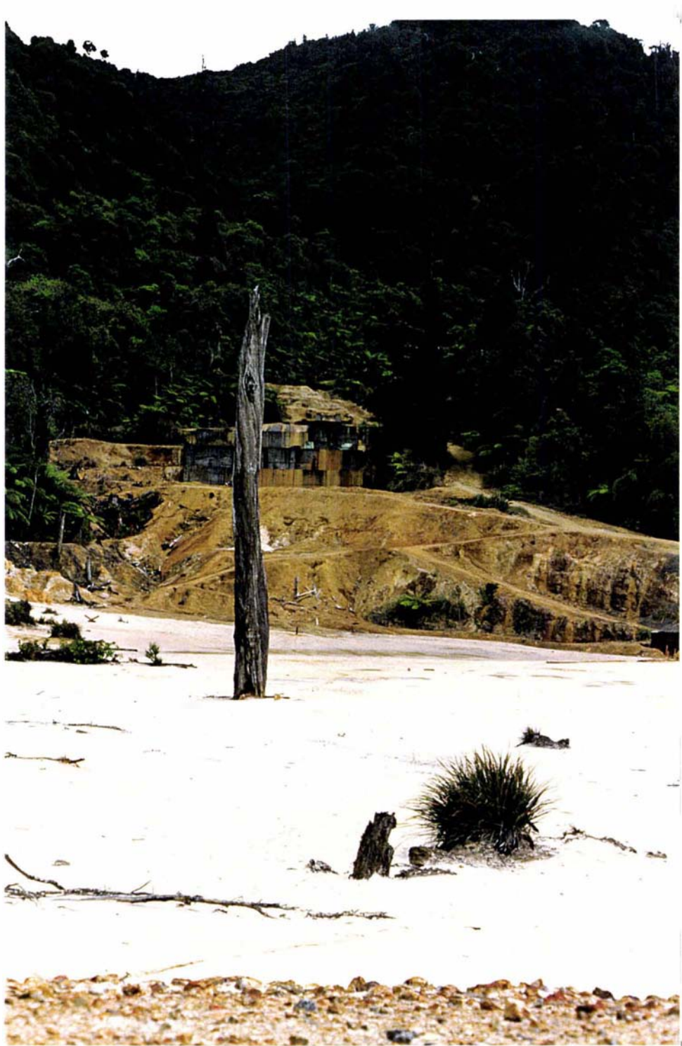
Plate 2.2 The Tui tailings dam and surrounding vegetation. The mine adits are located in dense bush in the top centre and left-hand-side of the photograph. (August 1993).
