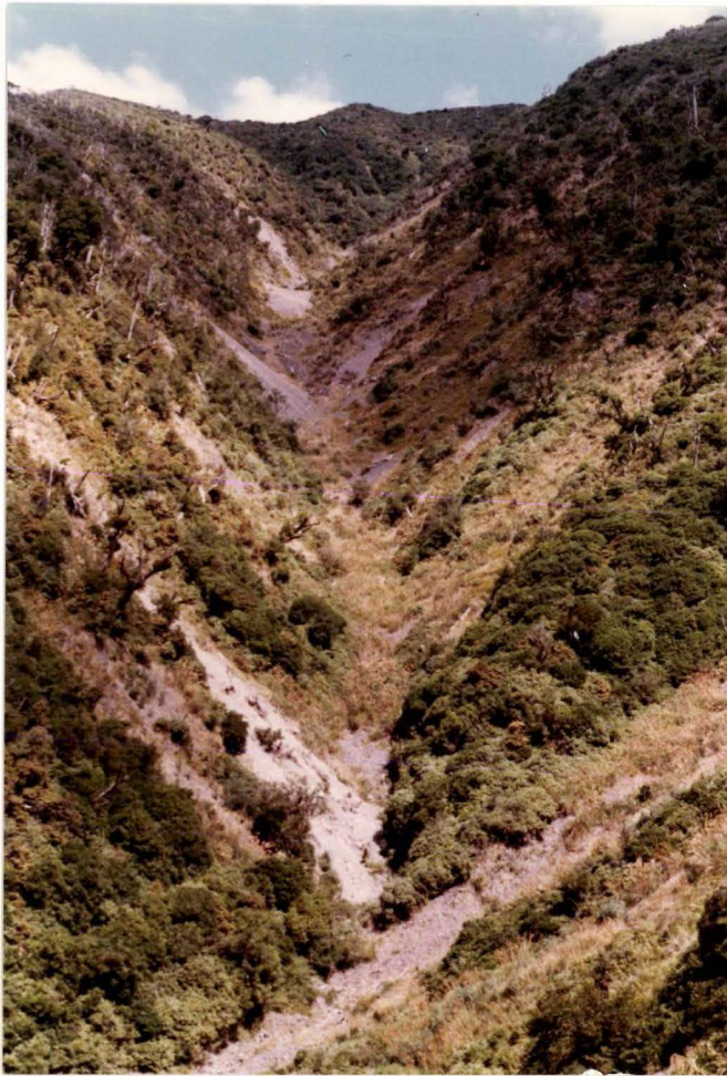
Fig. 11: Gully erosion in Car Park Creek (the vegetation is in a range of seral stages, being largely controlled by the erosion processes ).
