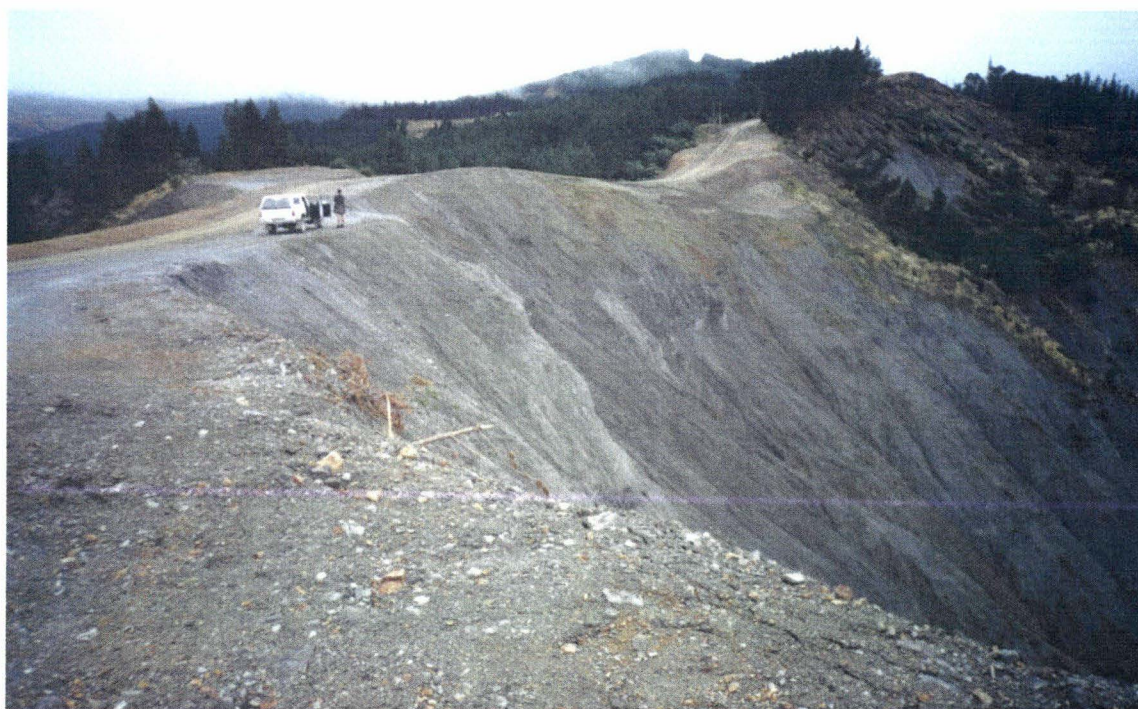
Plate 1.10.1 The ridge saddle at the head of the Tarndale Gully complex. This road separates the Mangatu (left) and Tarndale (right) gullies, continuous collapsing has meant that the road is now closed to most traffic (photo: M. A. D'Ath , 2000).
