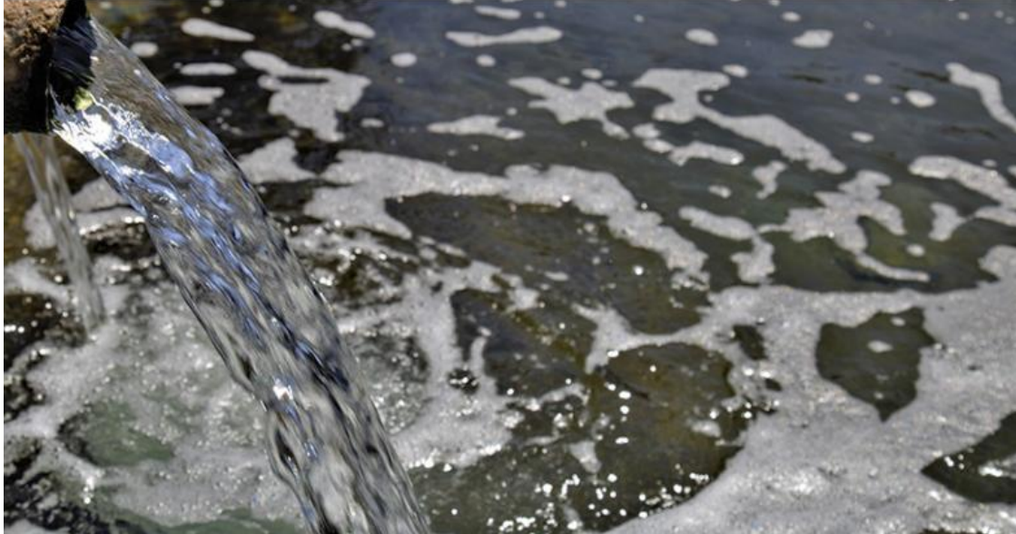
Figure 1.5. Rejected water from a small-scale desalination plant from one of the farms and which affects both the soil and the underlying groundwaters.
