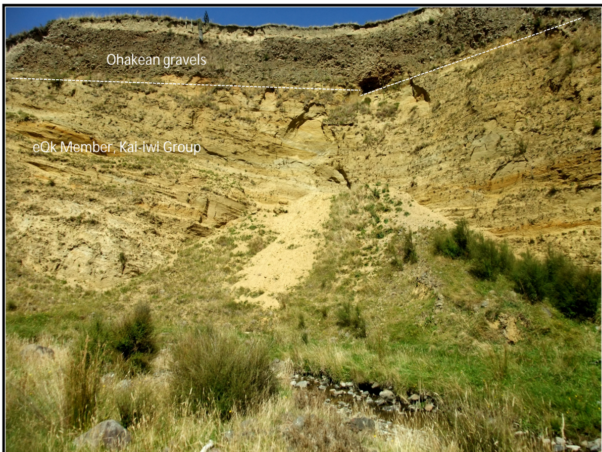
Fig 1.7: Horizontal Ohakean gravels forming angular unconformity with underlying eQk Member, Kai-iwi Group dipping 15^{\circ} @280 (NW). Maungatukurangi Stream, Broadlands Station, Pohangina Valley (WGS84 40^{\circ}15'00.75''S , 175^{\circ}47'46.95''E , elev 133 m).
