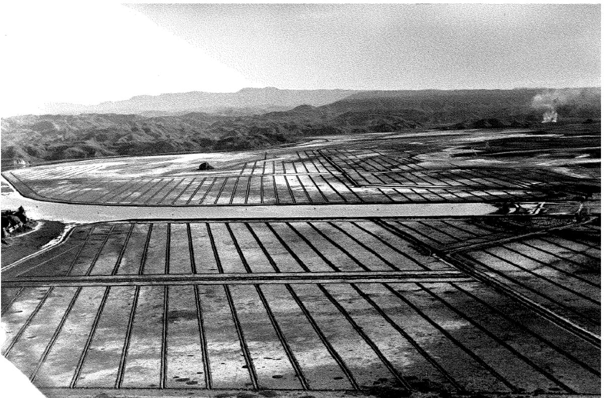
Figure 2.9: Land reclamation works adjacent to Ahuriri Estuary, circa 1936 (Parsons, 1992).
