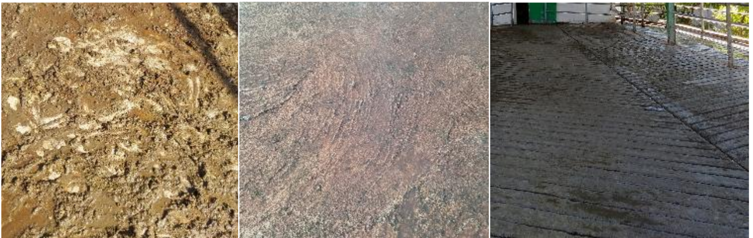
Figure 3.2. Different surface quality scores in parlour holding area- left: score 1: a smooth surface with potential chance of slipping; middle: score 2; non-grooved surface, but rough enough to avoid slipping; right: score 3; grooved concrete or rubber mats where chances of slipping are low
