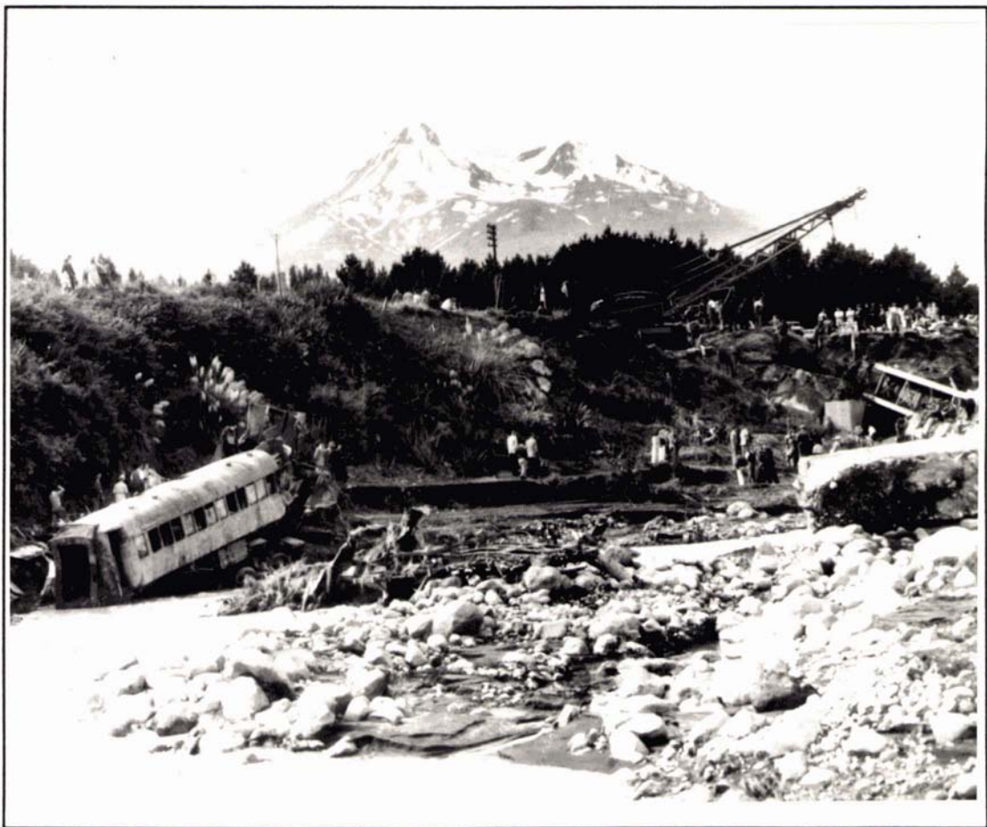
Plate 8.2 The scene at Tangiwai following the Christmas 1953 Tangiwai Disaster. Although the carriages in this photograph remained close to the bridge, another was carried nearly 3 km downstream by the lahar. The pile lying on the low terrace in the foreground of the photograph weighs 125 tons, and was carried 70 m downstream by the lahar.
