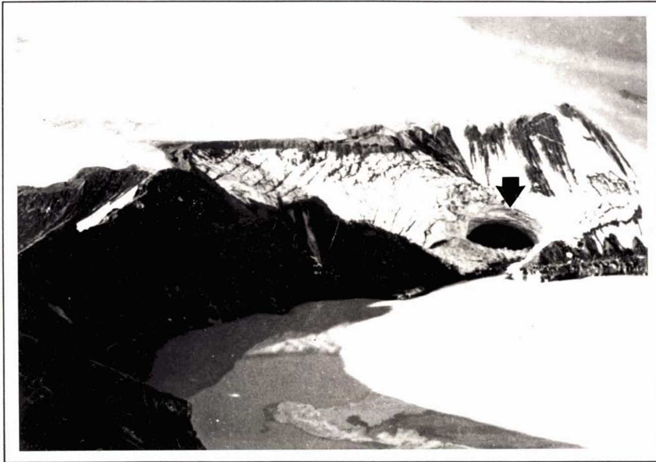
Plate 8.4 Crater Lake in December, 1953, following the Tangiwai Disaster. The hole in the ice and tephra barrier is marked by an arrow. Note also the top of another hole immediately to the left, which has been mostly buried by fallen ice. The lake level fell by about 9 m, releasing 1.6 \times 10^6 m 3 of water.
