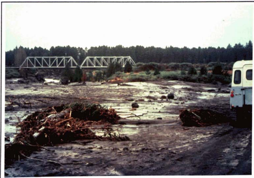
Plate 8.5 Tangiwai following the 1975 lahar, looking downstream towards the replaced railway bridge. The discharge and total volume for this event was similar to the 1953 lahar, but the new railway bridge survived. Photograph courtesy of T. Hurst, Department of Geological and Nuclear Sciences, Wairakei.
