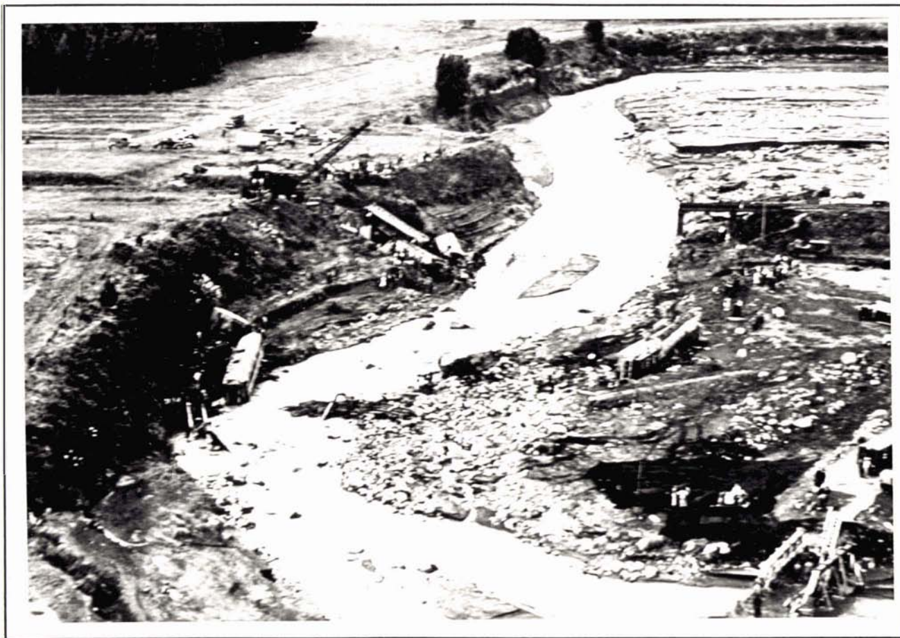
Plate 8.3 Tangiwai, December 1953, looking upstream towards the railway bridge. The lahar swept across the terrace in the right of this photograph, and across the road bridge in the bottom of the photograph, below the rail bridge.
