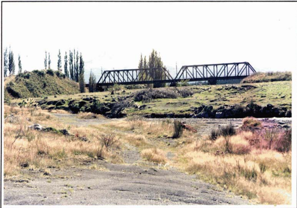
Plate 8.1 Tangiwai railway bridge with Mount Ruapehu in the background, April 1990.
