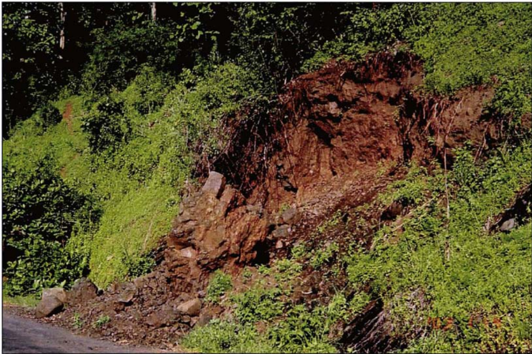
Figure 2-17 Small land slide on the roadside
