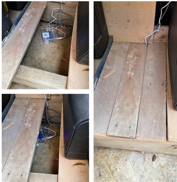
Figure H-4. Sensor installed on a concrete floor in a storeroom, aligned to true north, and secured with wooden planks to avoid disturbances.
