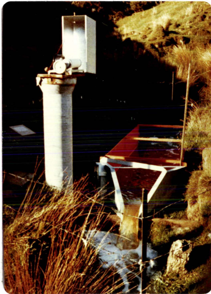
Fig. 2.6 H-S flume and Stevens F-type flow recorder operating on the stream draining the 6-ha catchment.
