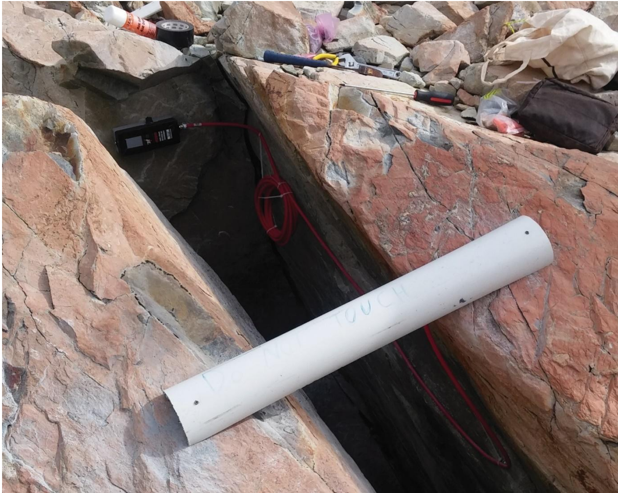
Figure 4-5: Crackmeter adjacent to Mueller Hut. The crackmeter lies under the protective pipe with the logging equipment connected to the wall of the fracture above the crackmeter.
