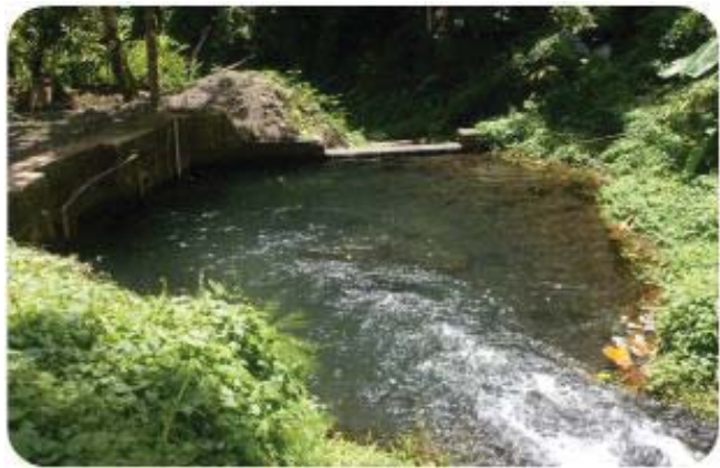
Figure 16. SWA water intake downstream from STN4
