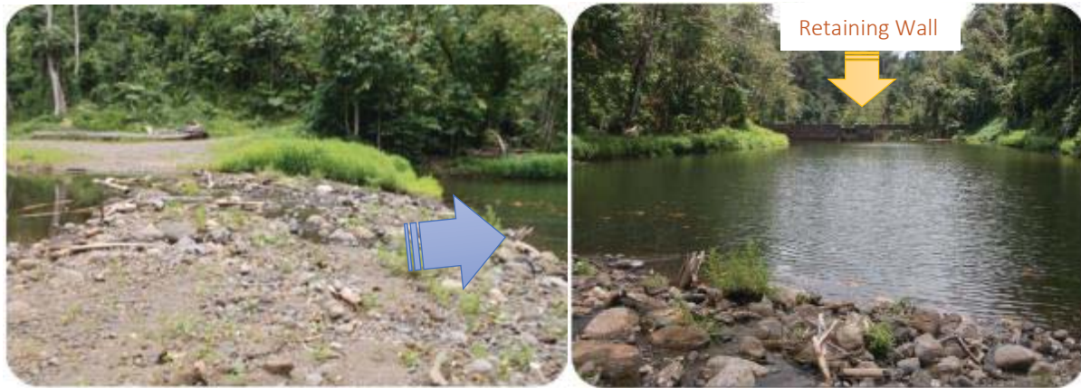
20 (a) Road track crossing Fuluasou River
