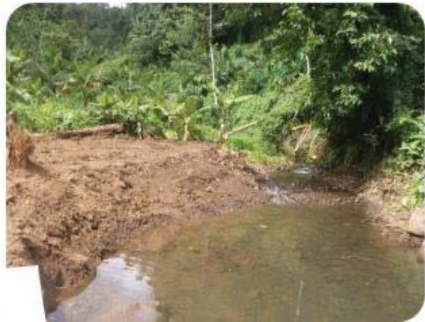
Figure 38. Chinese 2 where river water flows into the intake
