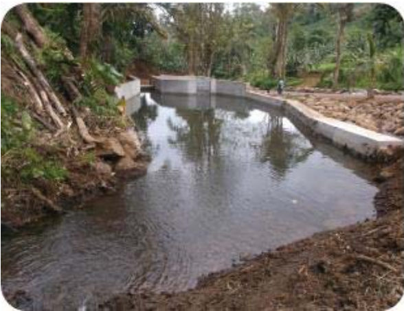
Figure 37. Chinese 2 water intake view from upstream
