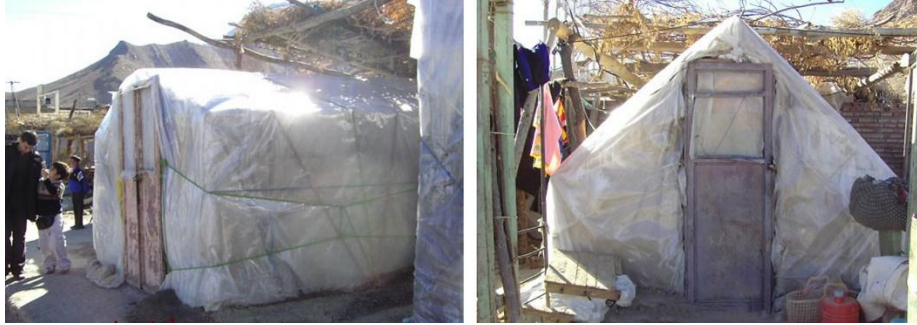
Figure 6.2. The tents were covered with plastic sheets by the users to endure the cold winter
