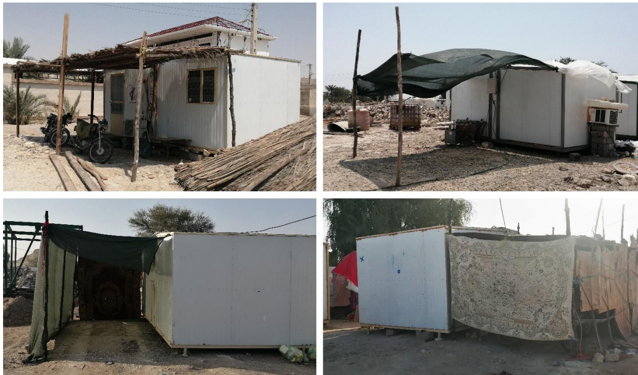
Figure 5.6. Informal extensions of the temporary housing units to overcome the space shortage and climate incompatibilities, canopies are made of fabric or palm leaves.
