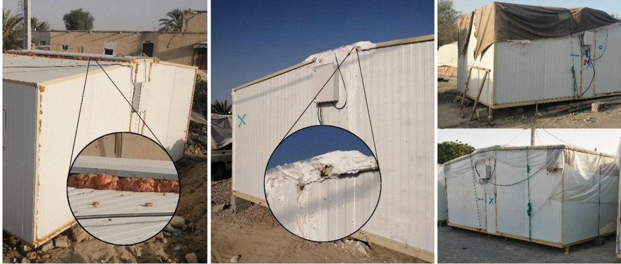
Figure 5.5. Sealing done by displaced people. Left: polyurethane foam. Middle: plaster mortar. Right: plastic covering.
