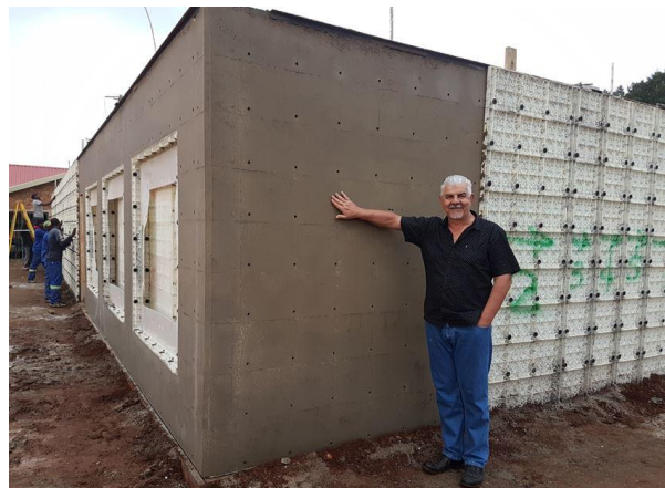
Figure 2.5. Moladi formwork, a cast-in-place structural system
