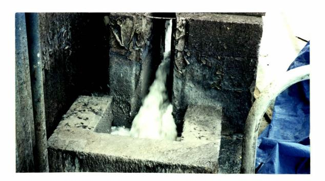
Plate 3.2 Discharge of untreated tannery effluent with high Cr concentration (3200 mg/L) into a public sewage system, from a tannery in Wanganui.
