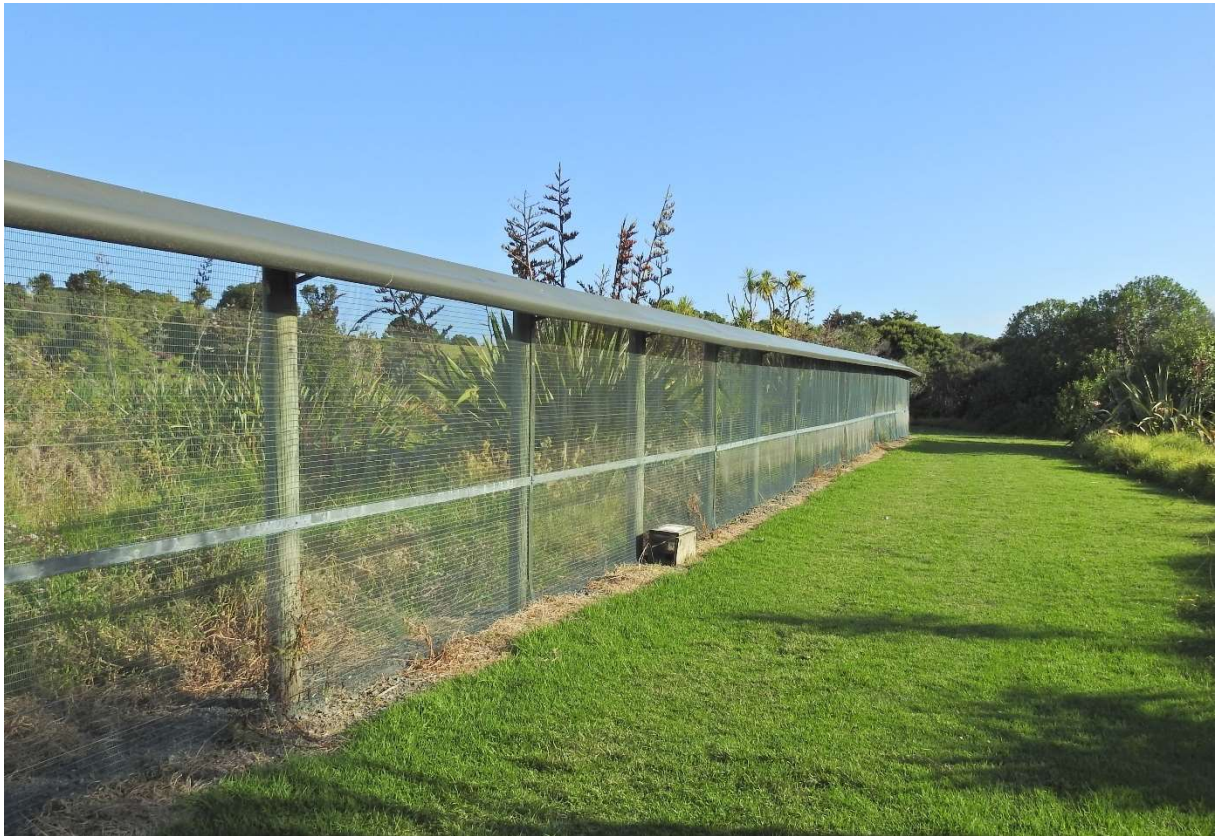
Figure 2.7: Photograph of the multi-species pest proof fence at Shakespear Open Sanctuary. Photo credit: Hayden Pye.
