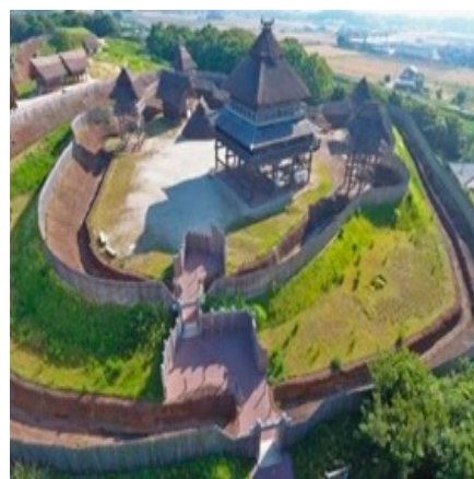
Figure 2. Key-shaped entrance of Kitanaikaku. Source: the Yoshinogari Historical Park's official website ( https://www.yoshinogari.jp ).
